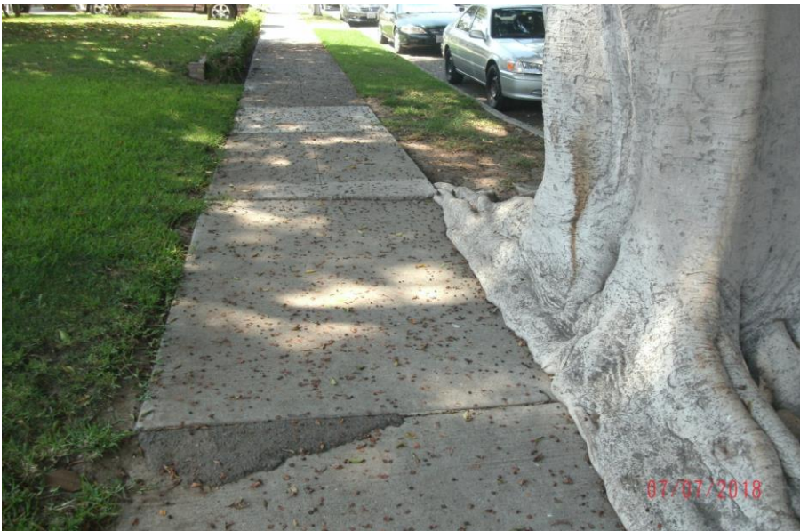
Tree with root intrusion and sidewalk damage
