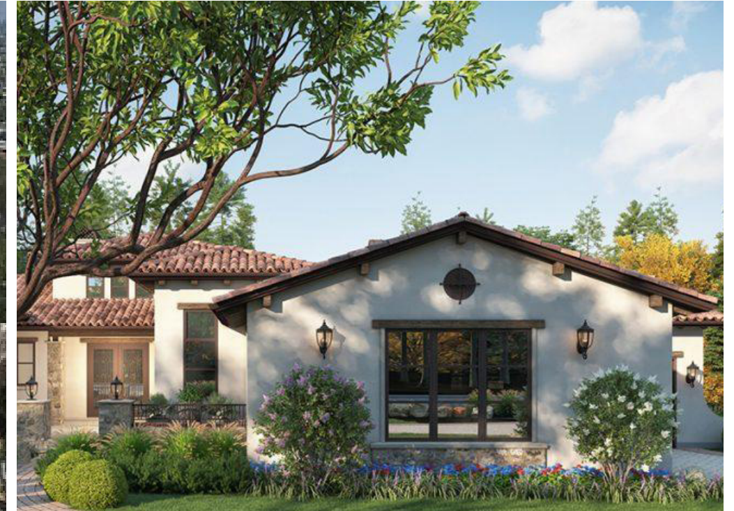
MINIMAL EAVES WITH EXPOSED RAFTERS
