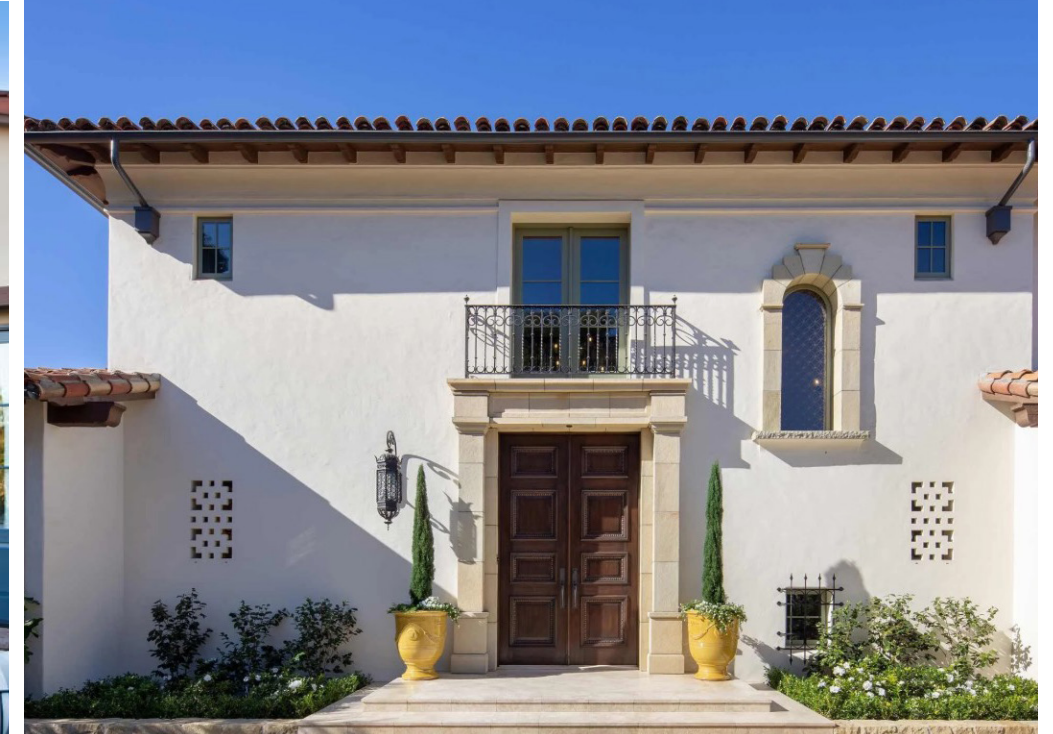
OVERHANGING EAVES + EXPOSED RAFTERS
