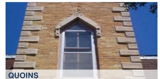
QUOINS Typically made of stone or contrasting brick, quoins are cornerstones that visually reinforce the edges of a building
