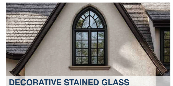
DECORATIVE STAINED GLASS Small panes of glass joined by slender strips, often arranged in diamond or rectangular patterns
