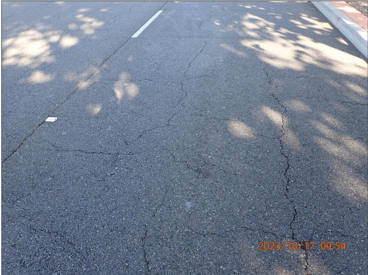
Figure 11 – 2023 Tight/Narrow Cracks
