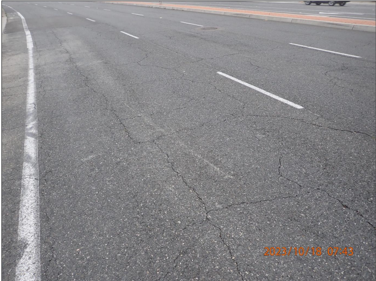
Figure 3 – 2023 Tight/Narrow Cracks
