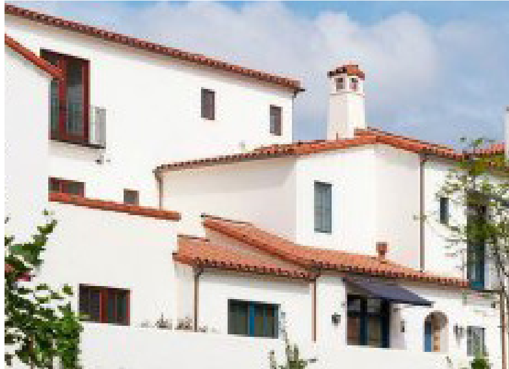
RED CLAY/CONCRETE TILE ROOF
