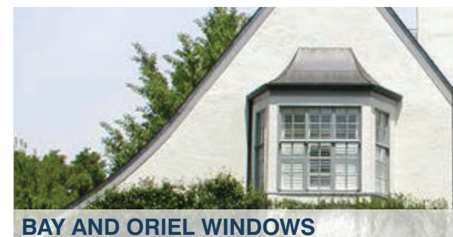
BAY AND ORIEL WINDOWS Projecting windows that add depth, light and visual interest to the facade
