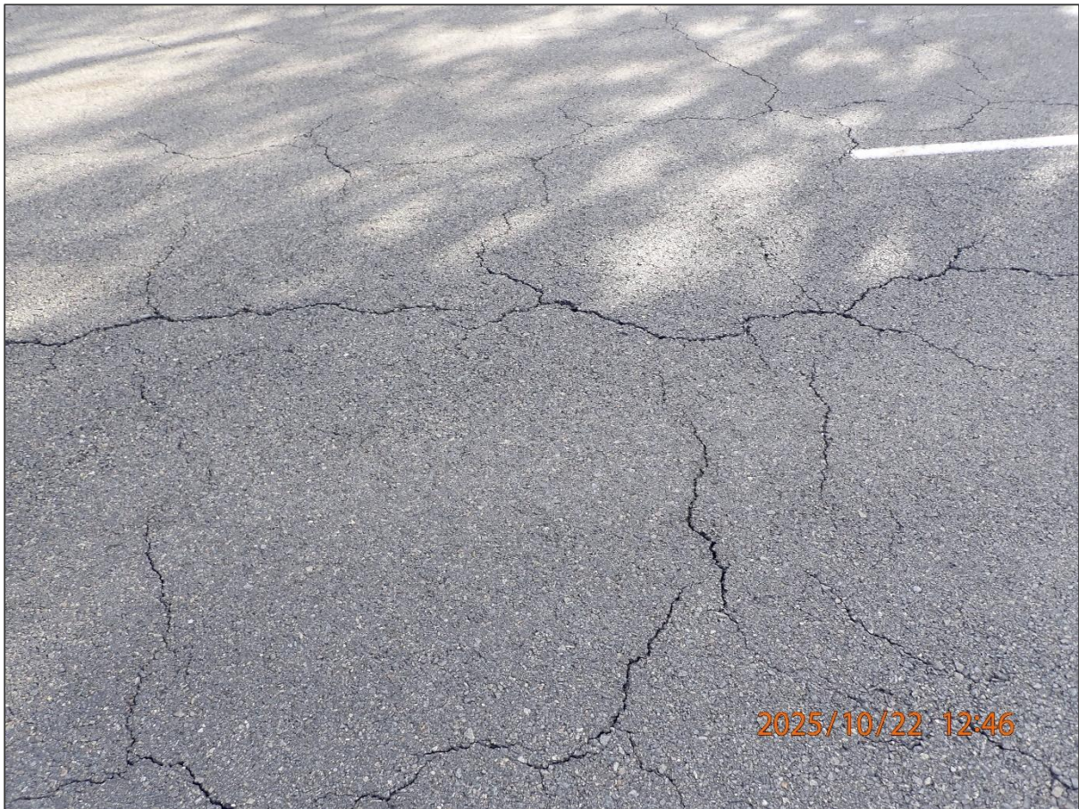
Figure 12 – 2025 Wide Cracks
