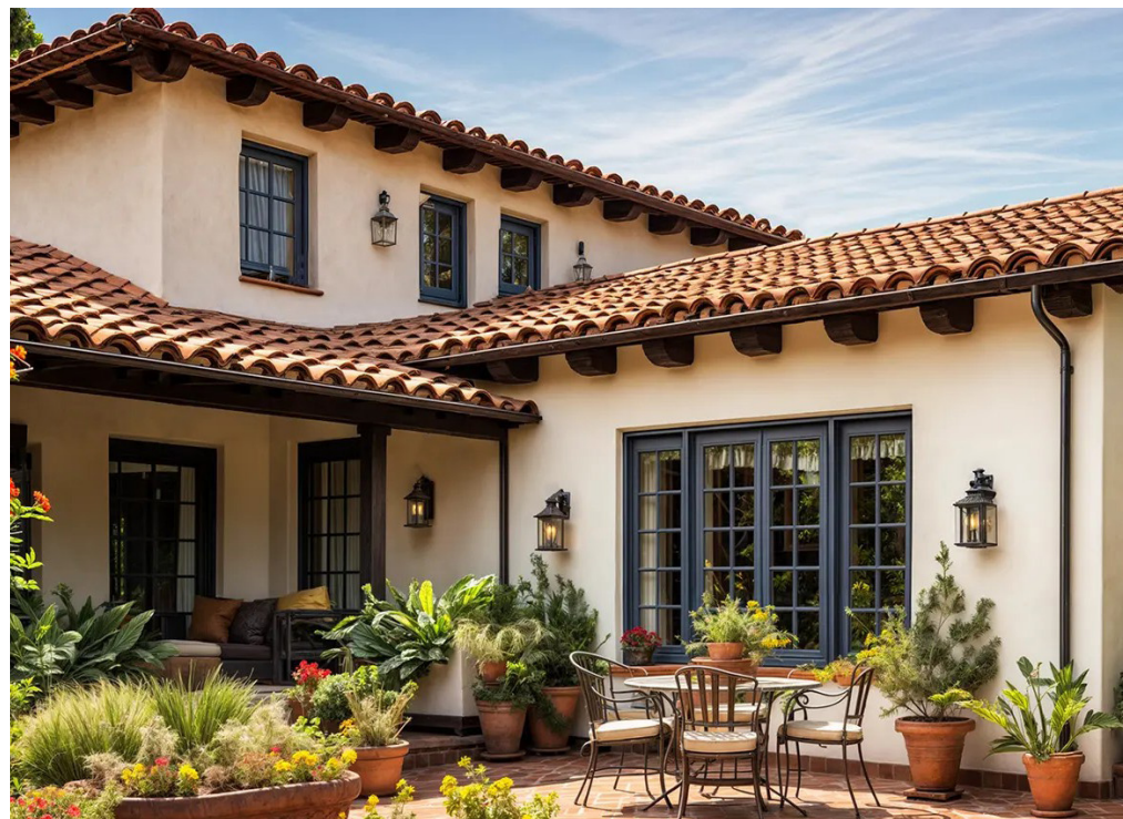
SHED ROOF OVER PORCH
