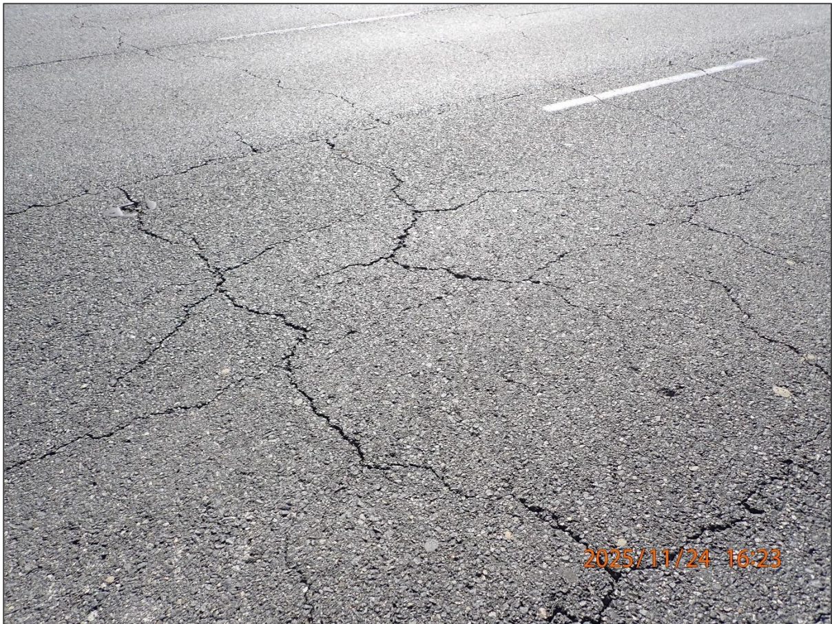
Figure 4 – 2025 Wide Cracks
