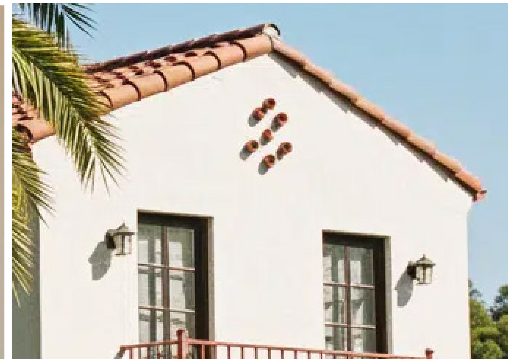
RED CLAY/CONCRETE TILE VENTS
