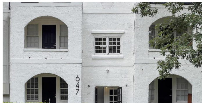
Sand-finished cement plaster on balcony, porch
