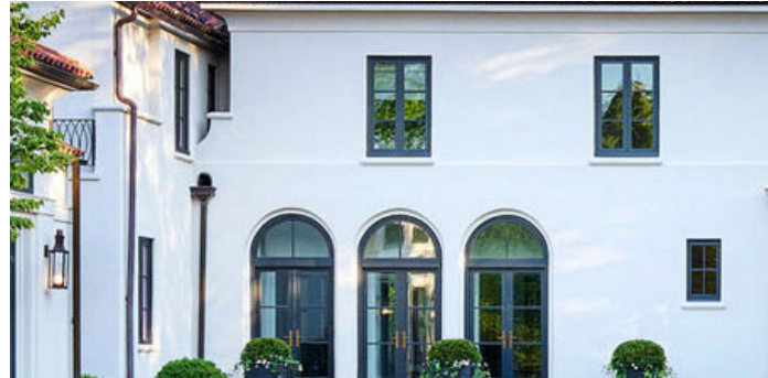
Stucco on exterior walls
