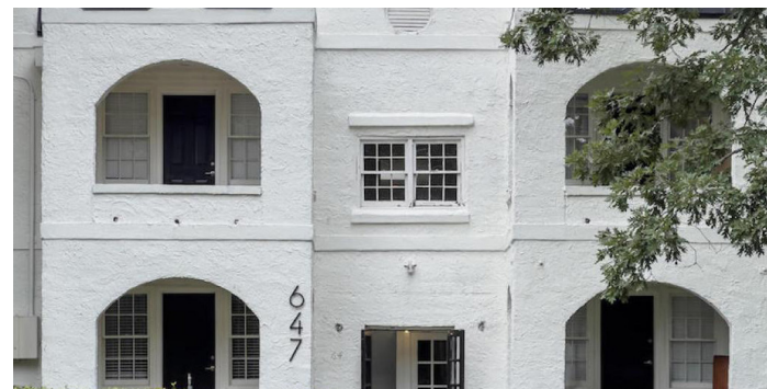
Sand-finished cement plaster on balcony, porch
