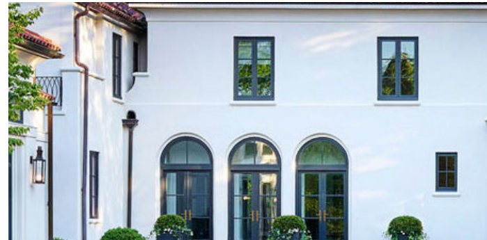
Stucco on exterior walls
